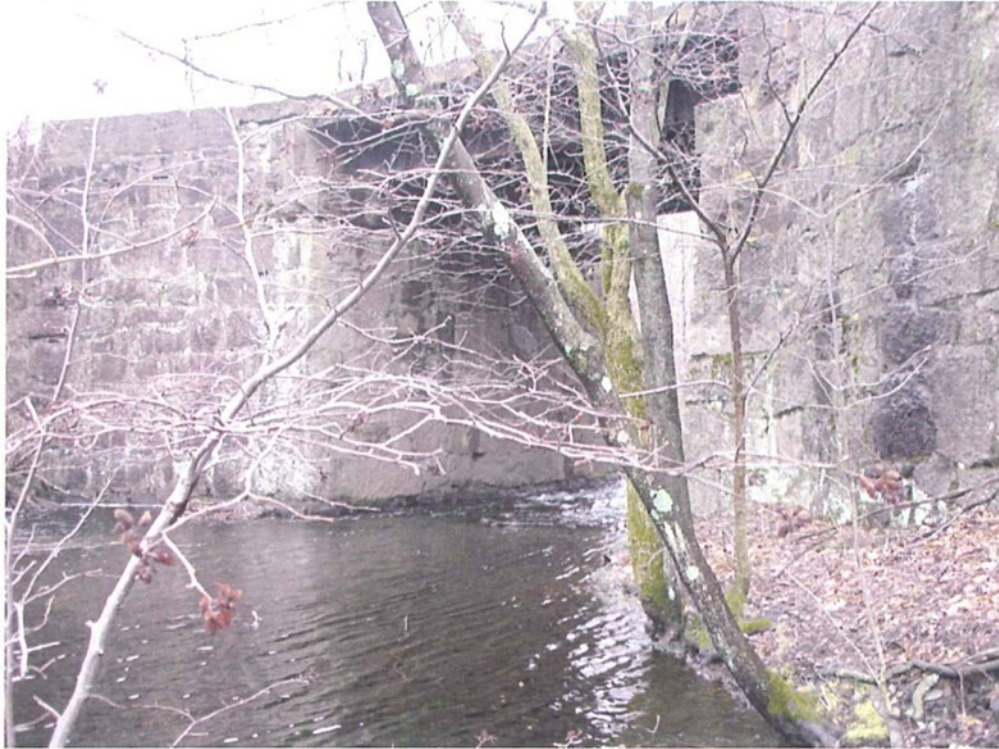
Photograph No.3: Railroad Bridge (MM 1.013)
